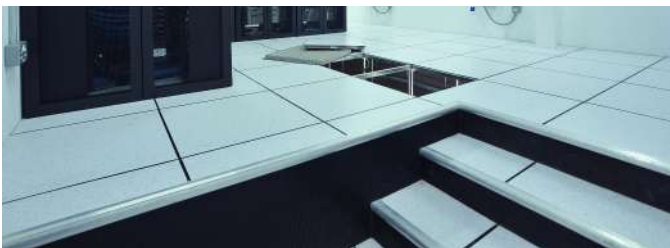
Raised floor steps and fascia
