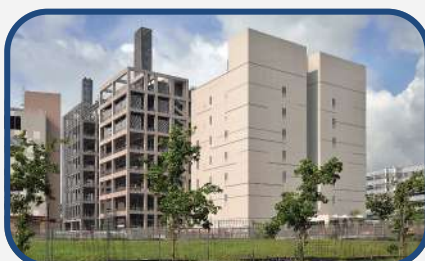
Data Centre at Jurong
