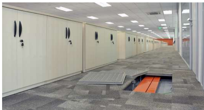
Completed office access floor system - Carpet Finish
