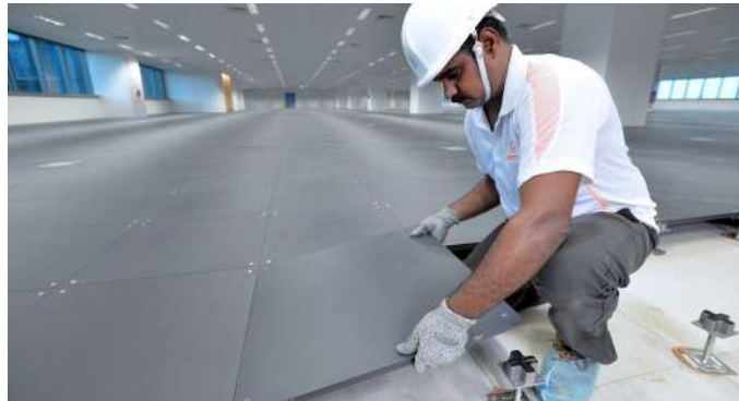
Installation of full access floor panels
