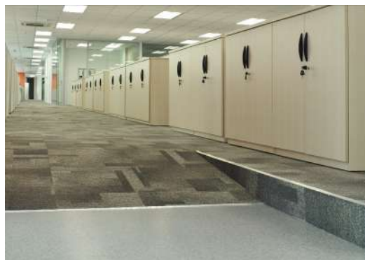
Ramp with carpet finishes (finishes by others)
