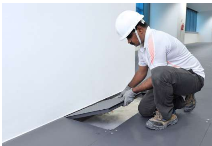
Installation of cut panels at perimeter
