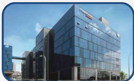
Research & Commercial Building at Depot Road
