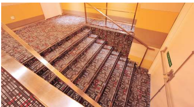
Raised floor steps and fascia
